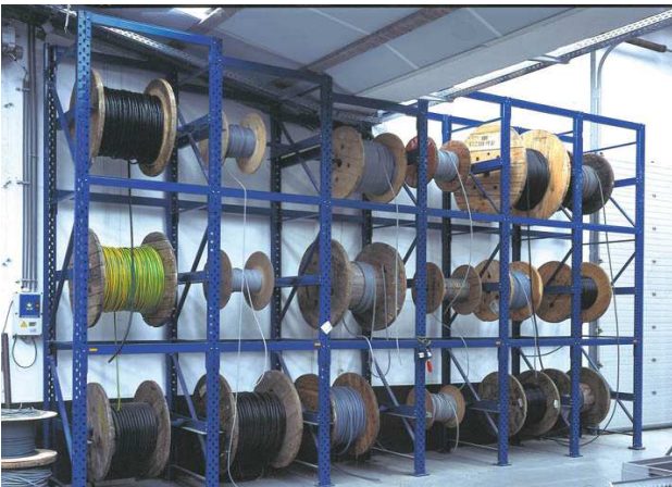
▼ Cable drum storage.
