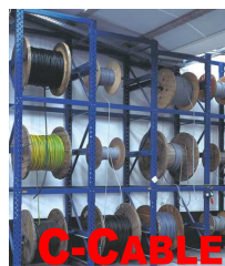
C-CABLE Cable drum storage
